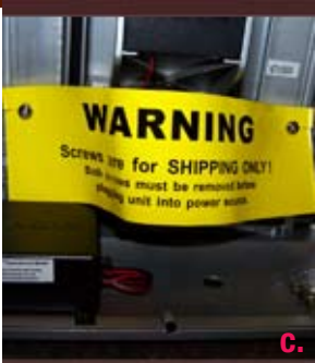
1c. Completely remove two shipping screws indicated by the yellow warning label.
